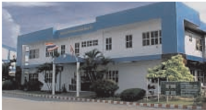
P.C.B. Center factory, Chonburi, Thailand
